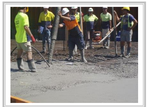
Figure 2: Pouring the concrete containing Radmyx
